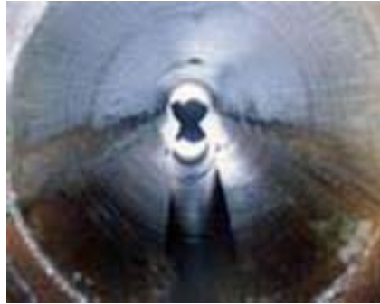
Clean Sewer Pipe
